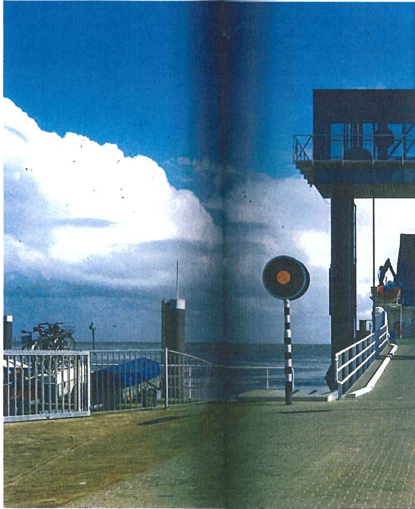
Landing stage structure
